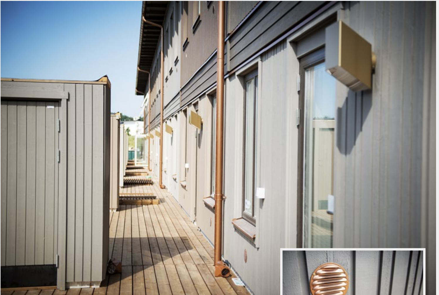
The nineteen Plusshus modules built in Barkarby west of Stockholm have acquired their own character due to individual colours and outdoor light fittings specially developed for the area.
