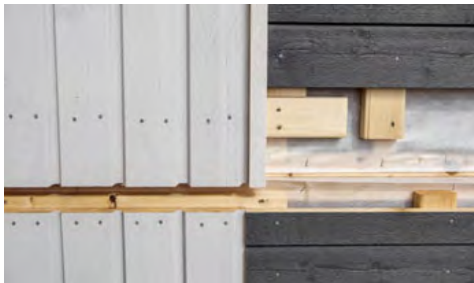
The timber beneath is hidden by pre-painted boards to give the facade the perfect finish.
