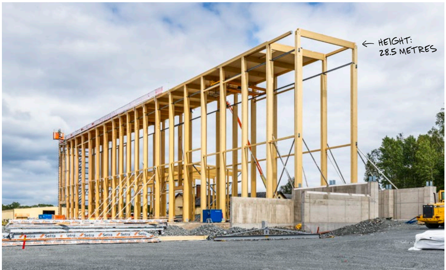
The glulam frame for the new facility in Hasselfors is Setra Långshyttan's biggest project so far.
