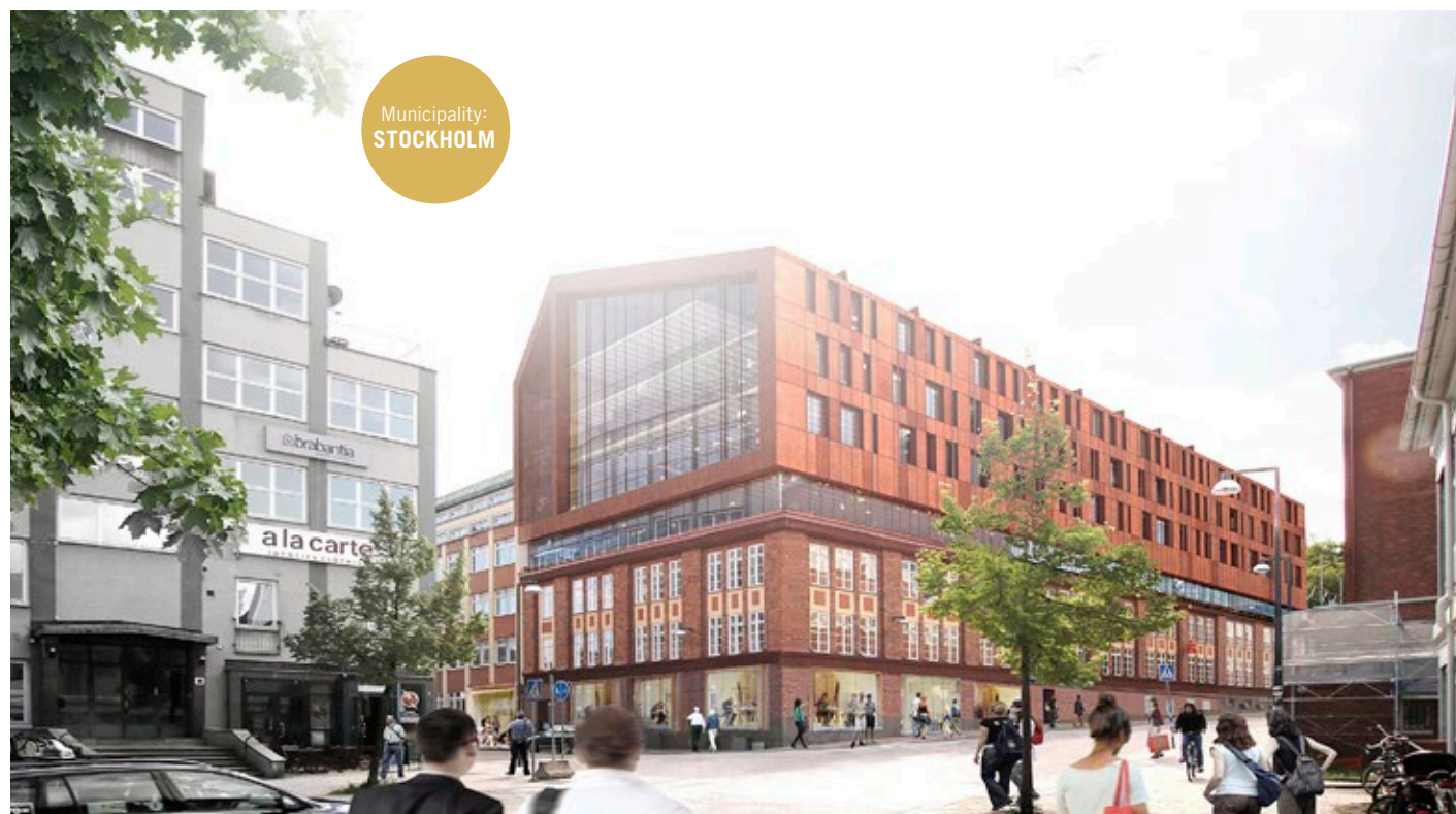
The lightness of wood has made it possible to add several floors of offices on top of Trikäfabriken, an old brick building in Hammarby Sjöstad. Architect: Tengbom
