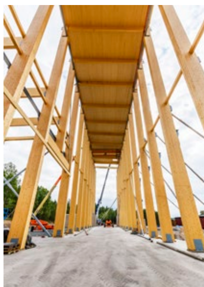
Although the design is complex, the process of assembling the glulam frame has proven a pleasant surprise for the workforce.
