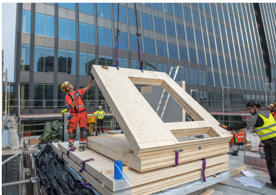
The deliveries are planned even before the factory begins producing the crosslam elements, so everything arrives in the right order.
