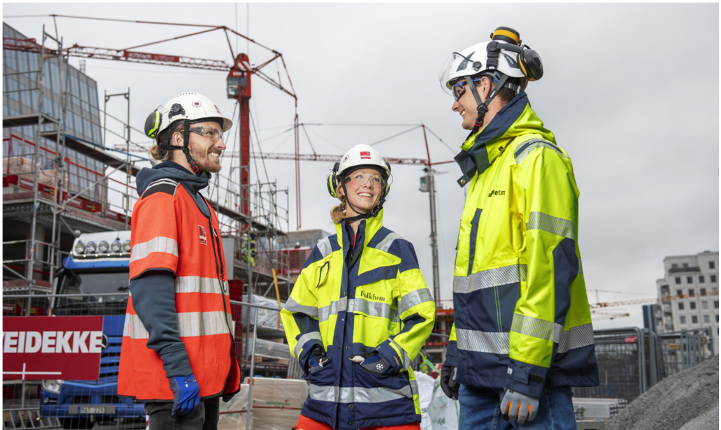
Jakob Tengvald, Project Manager Veidekke, Anna Ervast Öberg, Project Developer Folkhem and Emil Öbrink, Project Manager Setra are on site in Hagastaden, where Cederhusen's first building is now going up.
