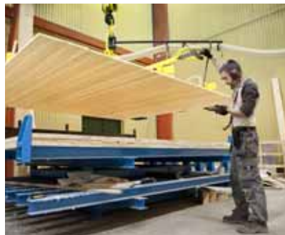
Plusshus’ wall element order leads to new working duties in the finishing unit.
