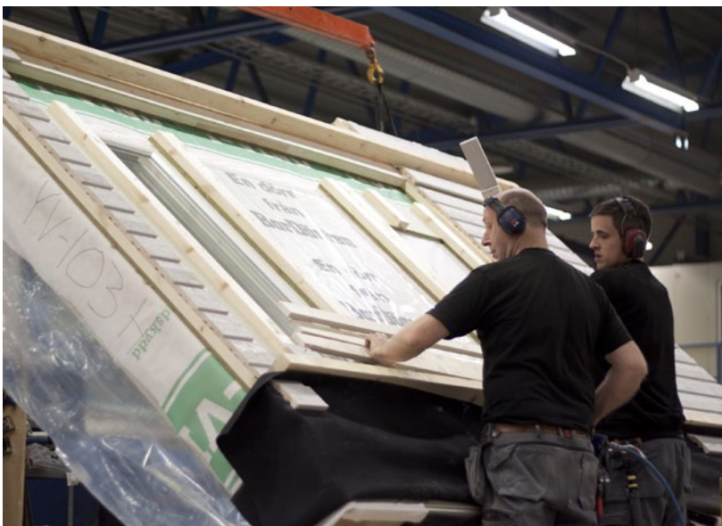
Employees at the Plusshus factory in Renholmen manufacture both house modules and box units.
