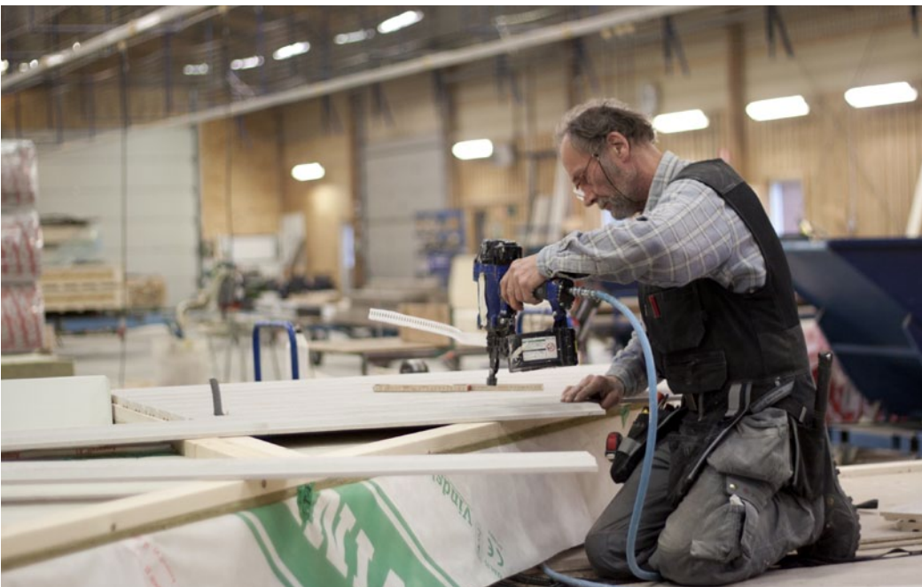
Box units are completed in a dry and safe environment. Here exterior cladding is being placed on a box unit for a terraced house.
