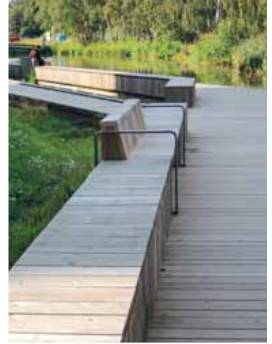
This beautiful, wooden-decked walkway, with cleverly recessed benches, goes along the water's edge in the new Annedal district on the border between Stockholm and Sundbyberg.
