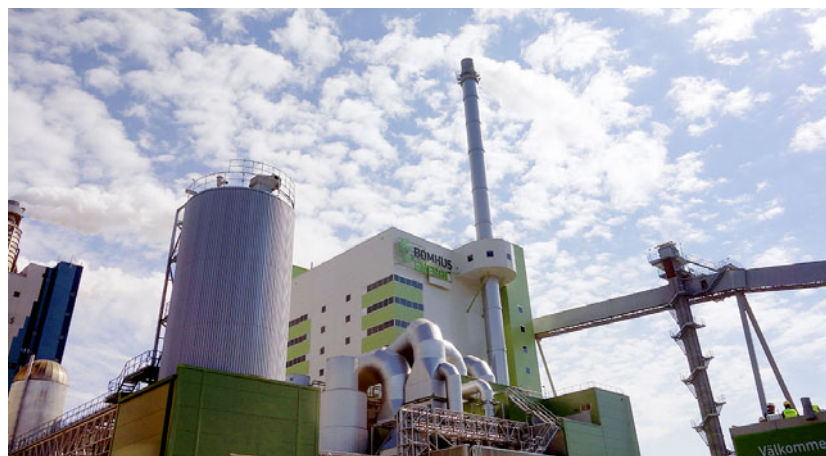
Bomhus Energi is an ultra-modern CHP plant which is supplied with fuel from its immediate neighbour Setra Kastet, among others.
