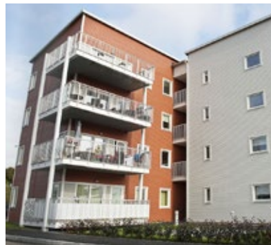
An apartment block in the Sâgen district in Knivsta north of Stockholm, delivered as modules from Plusshus.
