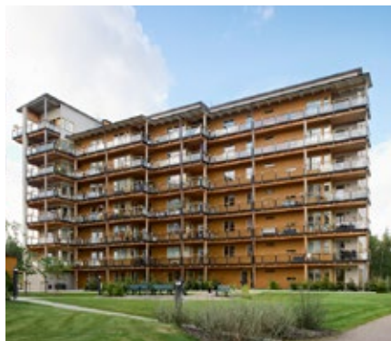
When construction was completed in 2009, Limnologen in Växjö was Sweden’s tallest newbuild apartment block with a wooden structural frame.
